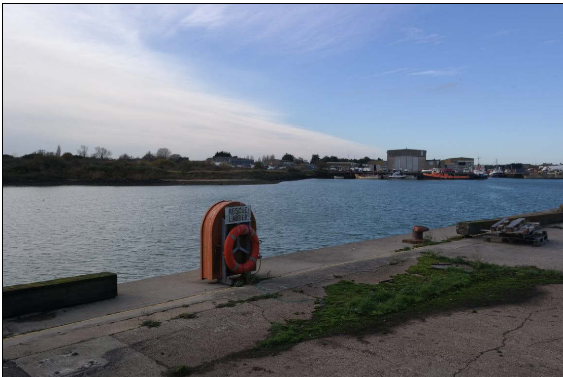
Plate 2: Lake Lothing, looking south west to reclaimed ground from area of option W4 and T3
